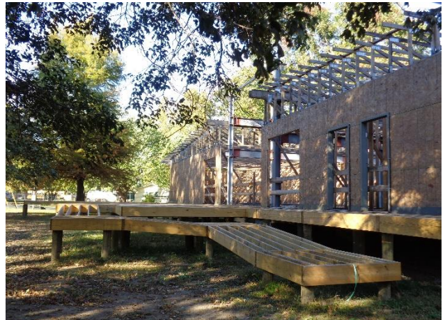
Construction of the interpretive visitor center at Reelfoot Lake.
