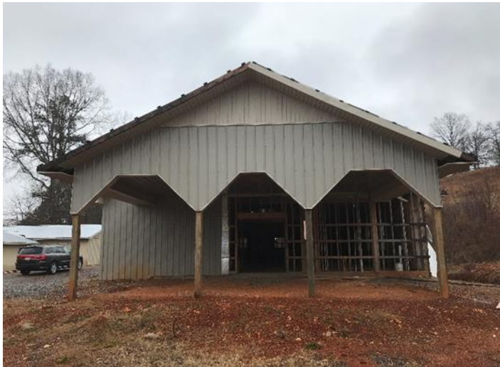
Peakland Baptist Church Rebuild
