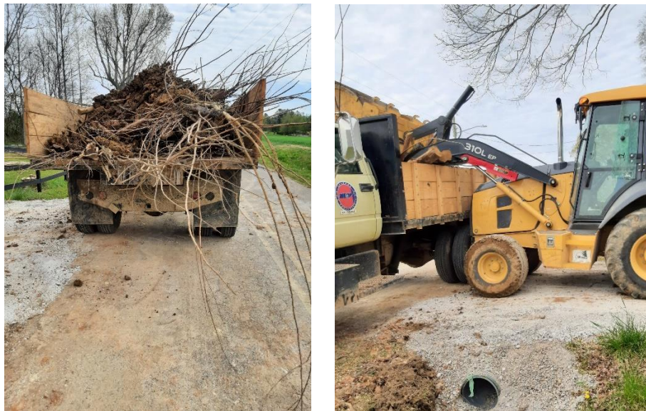
Debris removal from private property using city-owned equipment.
