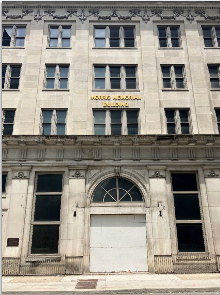
Exterior of the Morris Memorial Building located at 330 Dr. Martin Luther King Jr. Blvd. in Nashville, Tennessee
