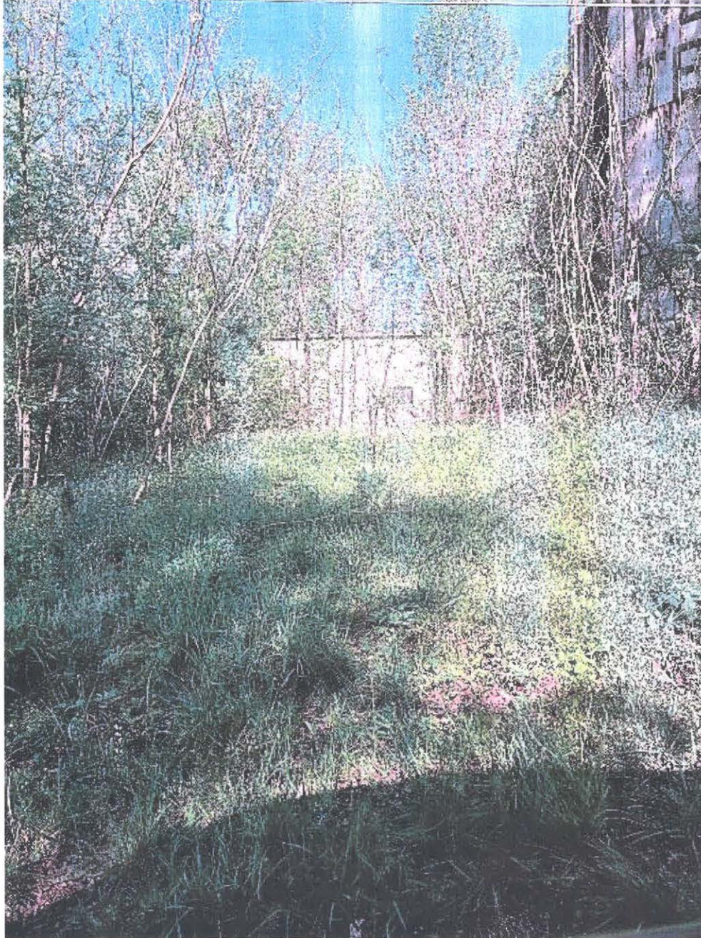
This is a picture of the abandoned and dilapidated water treatment plant. The plant is not functional, and all interior wiring and mechanicals have been removed.
