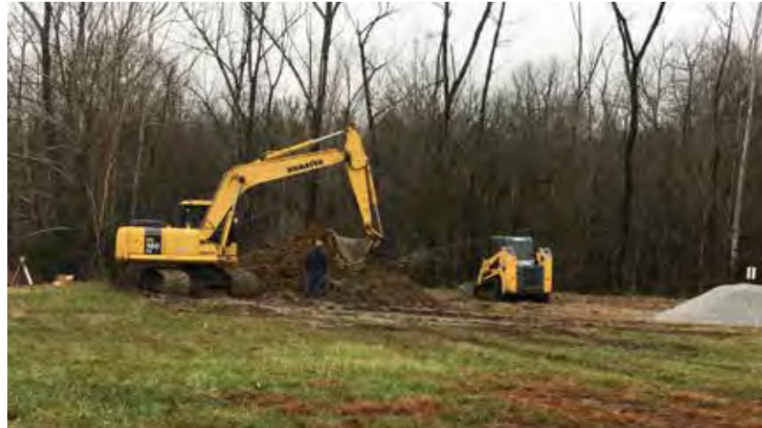
Village 1 Drainage Improvements
