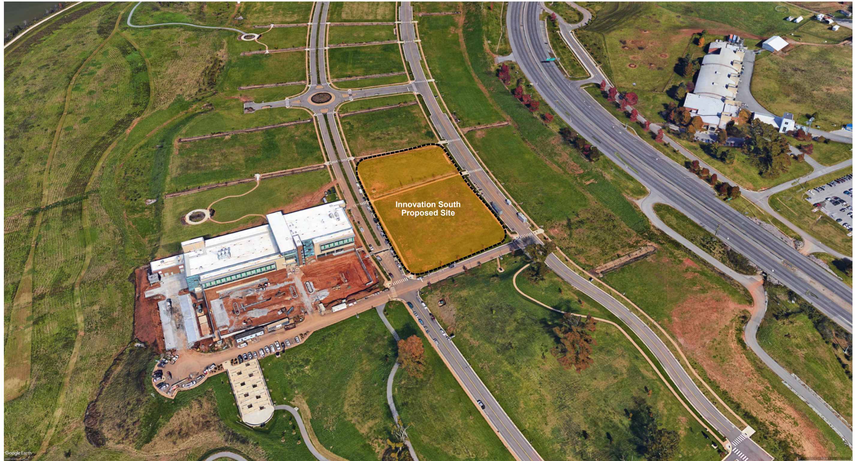
Site Aerial Showing JIAM Under Construction and the Innovation South Site
