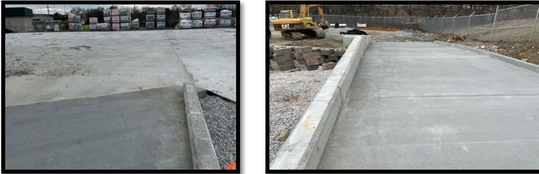
Photos of the construction project at the private business taken on January 26, 2023
